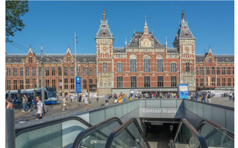
CS Amsterdam, (foto: Nikolai Kareneshev) Stationsbelevingsmonitor: 7,5 (2022)
