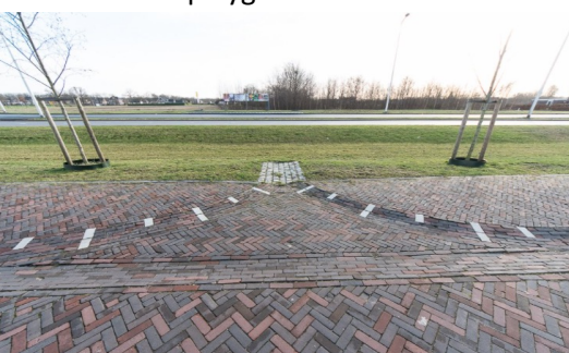
6 Gully free road to swale Almelo
